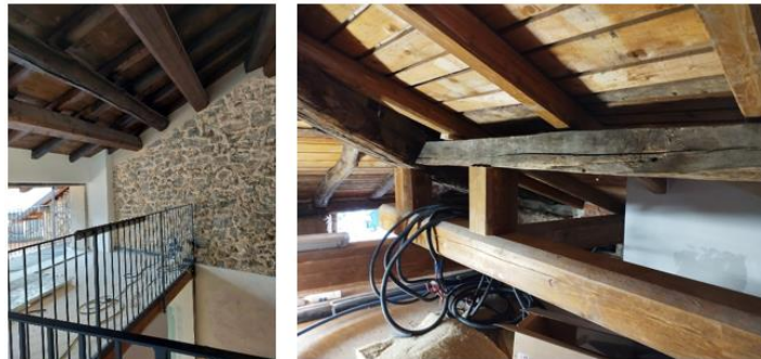
Figure 11 old and new wooden beams
