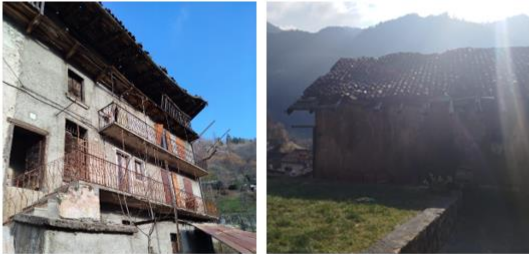
Figure 4 Facade and Back of Casa Renica
