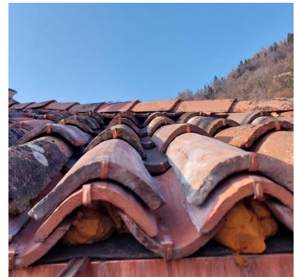
Figure 10 Copper hooks holding tiles
